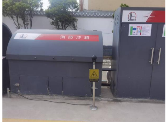
卸油口一侧消防沙箱及人体消除静电桩
